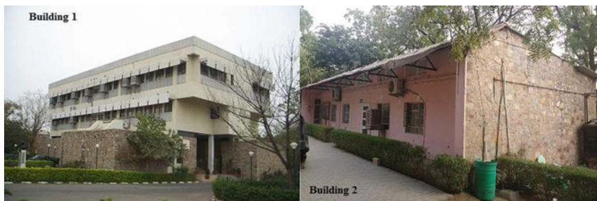
Fig. 3 Pictorial view of Building 1 and Building 2
