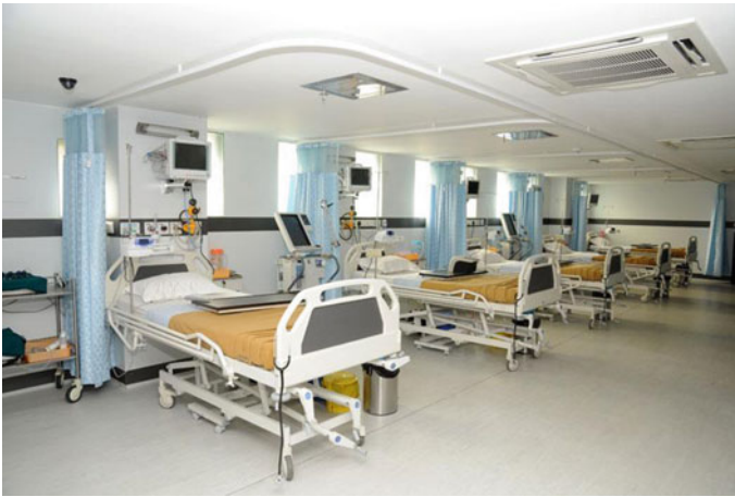
Fig. 6 Curtain partitioned ICUs with commercial air conditioners
